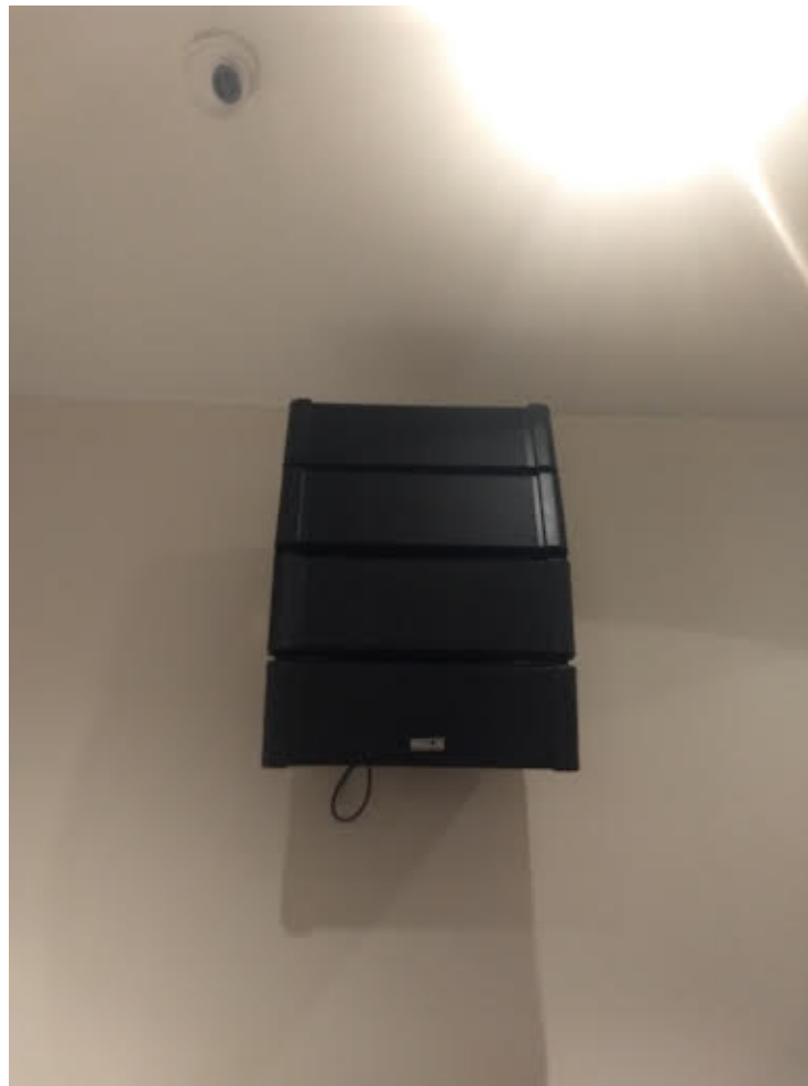
Figure 5.9: Line array speakers (four of them with different angles) Source: Author's Personal Collection
