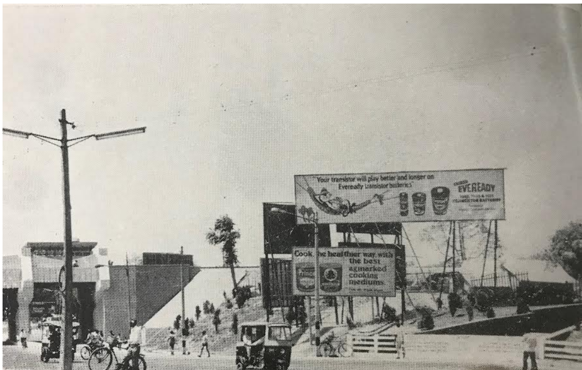
Figure 2.6: Photo #3 from DUAC report indicating hoardings as a menace to the cityscape (1974-5) Courtesy: IIMC Library
